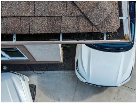
Figure 40. Detail 3 — Drainage / Gutters and Downspouts, North.
