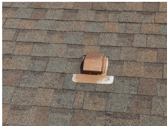
Figure 12. Detail 1 — Ventilation / Roof vent, Multiple.
