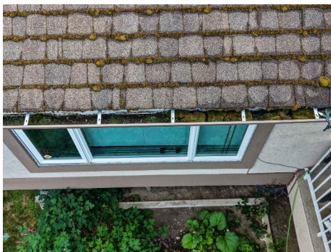
Figure 38. Detail 1 — Drainage / Gutters and Downspouts, North.
