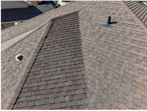
Figure 18. Detail 3 — Ridge / Valley / General observation, Multiple.
