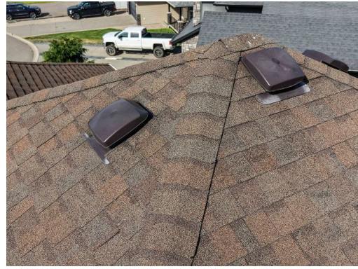
Figure 19. Detail 4 — Ridge / Valley / General observation, Multiple.
