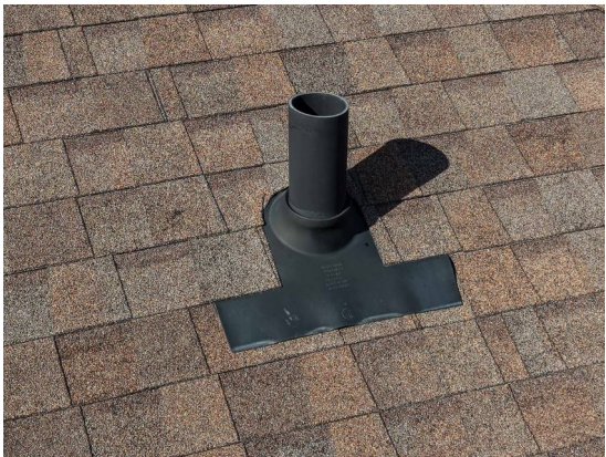
Figure 14. Detail 1 — Penetrations / Plumbing vent, South.
