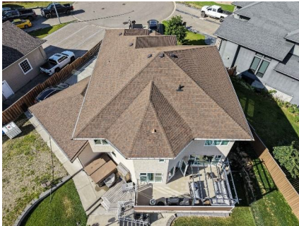
Figure 4. South roof overview.
