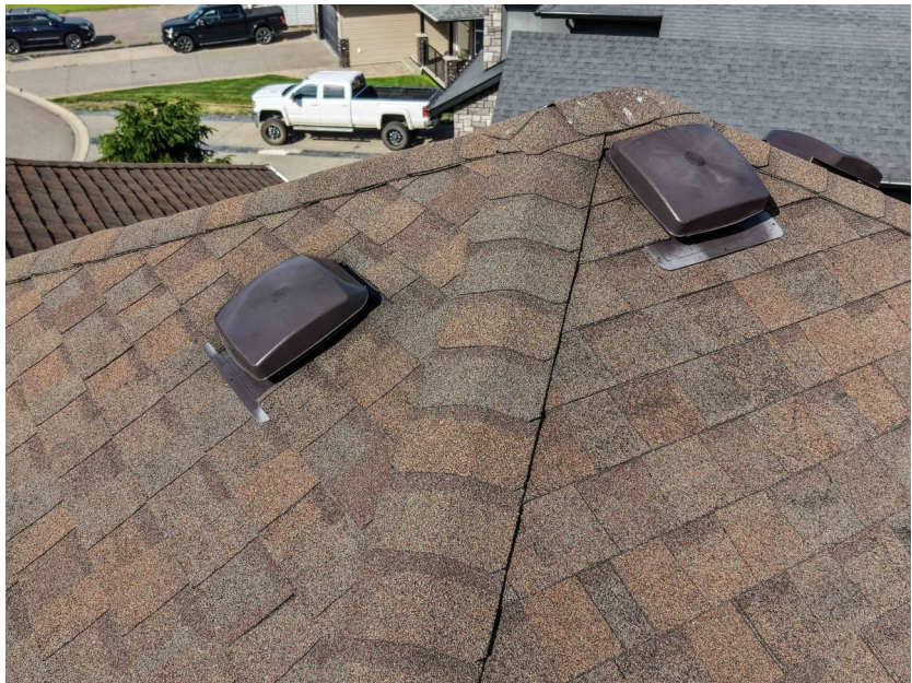
Figure 6. Overview — Ventilation / Roof vent, Multiple.
