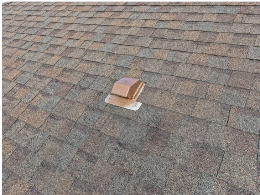
Figure 11. Overview — Ventilation / Roof vent, Multiple.
