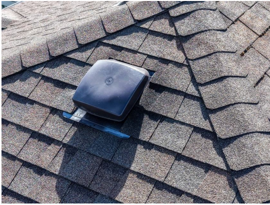
Figure 9. Detail 3 — Ventilation / Roof vent, Multiple.
