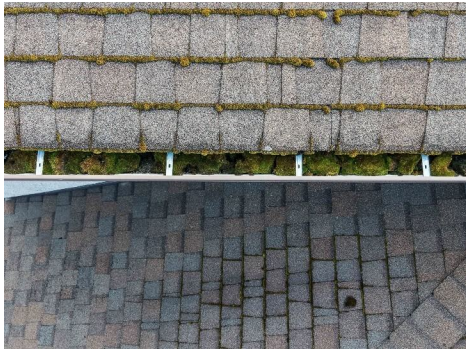
Figure 42. Detail 5 — Drainage / Gutters and Downspouts, North.
