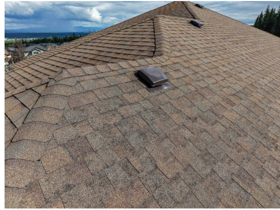
Figure 10. Detail 4 — Ventilation / Roof vent, Multiple.
