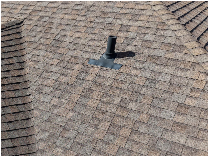
Figure 13. Overview — Penetrations / Plumbing vent, South.
