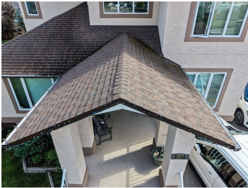
Figure 20. Detail 5 — Ridge / Valley / General observation, Multiple.
