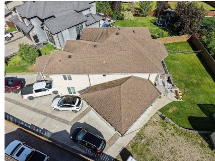
Figure 5. West roof overview.
