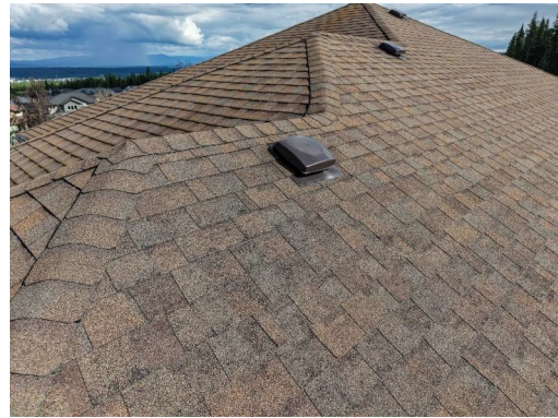
Figure 21. Detail 6 — Ridge / Valley / General observation, Multiple.
