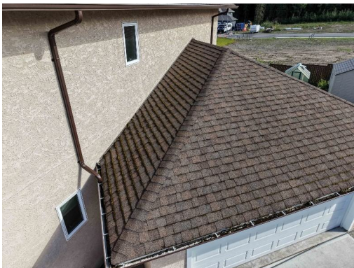
Figure 16. Detail 1 — Ridge / Valley / General observation, Multiple.
