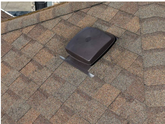
Figure 7. Detail 1 — Ventilation / Roof vent, Multiple.
