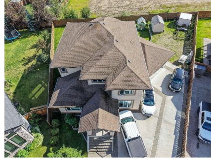
Figure 3. North roof overview.
