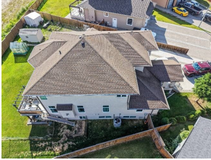
Figure 2. East roof overview.
