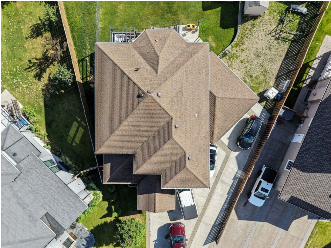
Figure 1. Roof vertical overview.
