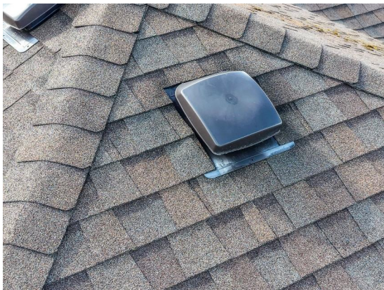
Figure 8. Detail 2 — Ventilation / Roof vent, Multiple.
